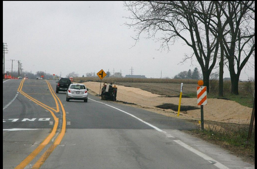
Crews place shoulder stone, striping and landscaping for the pavement widening on the Huntley Rd at Galligan Rd Intersection Improvement
